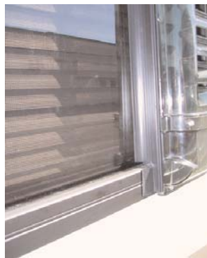
Cut Wiper Gasket FIG T
